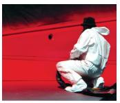
Sprayable Elastomers are a great solution for Plant Managers and Engineering Consultants who need to solve problems associated with abrasion, corrosion or erosion. They can be applied to old, worn out processing equipment as well as new equipment to assist in prolonging their operating service life.
