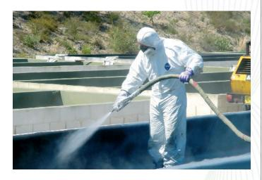
With the exception of one of the High Performance TDI Sprayable Elastomers, all the products within this range are 100% solids with Zero VOC; they are two component systems with a 1:1 mix ratio so are easy to use, with high-pressure spray equipment.
